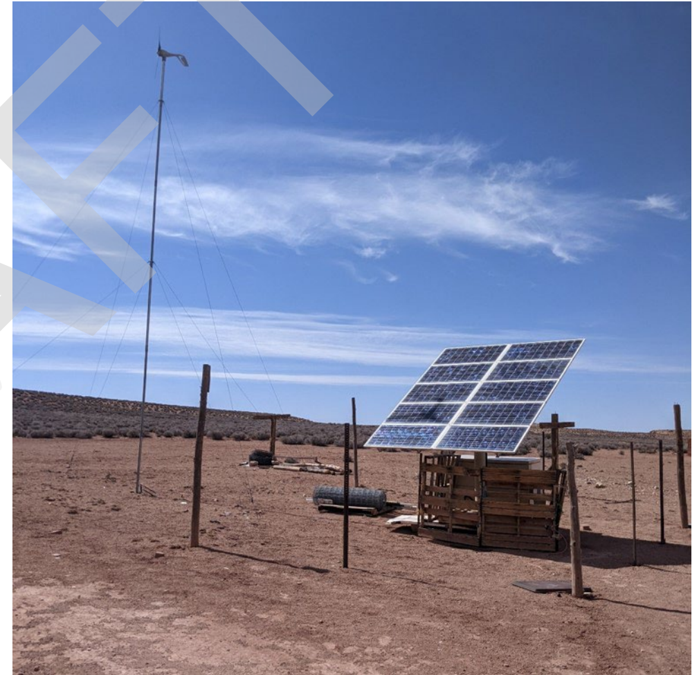
A solar-wind hybrid system like the systems NTUA provides their off-grid customers.
